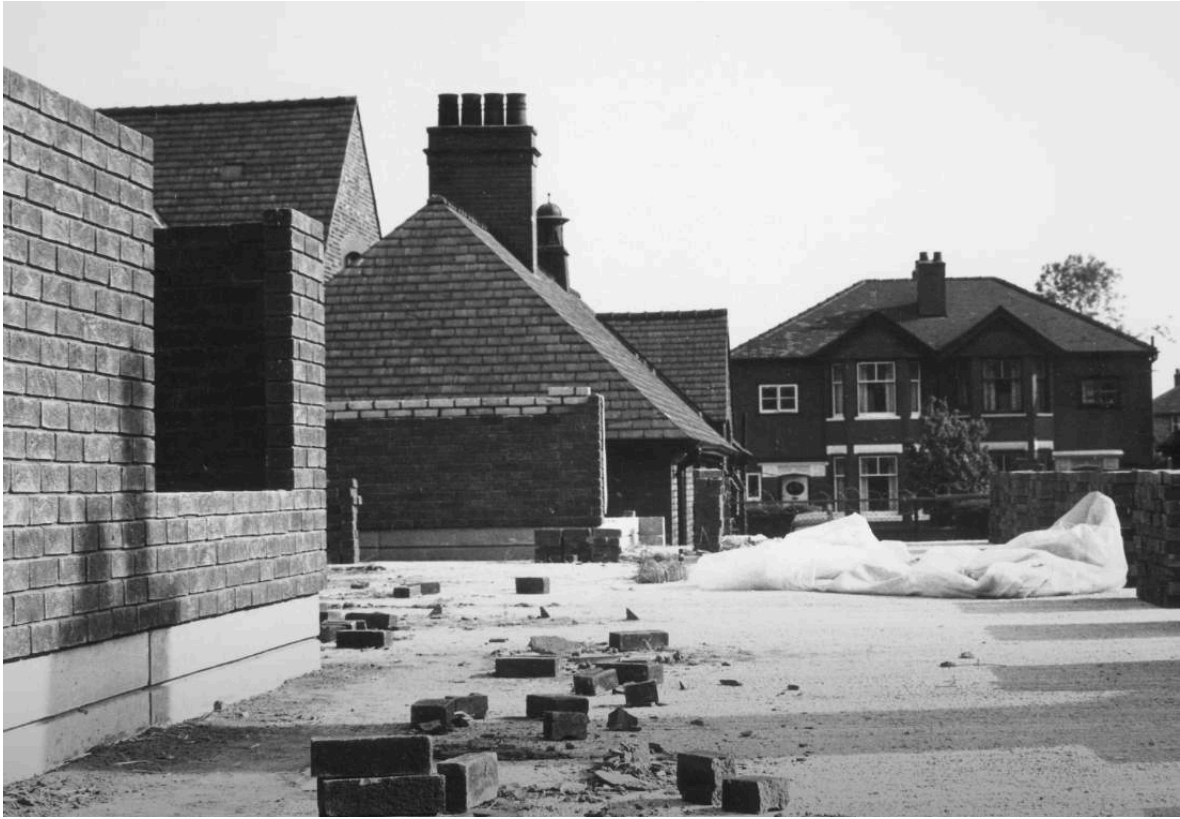
The work begins - looking towards Waller Avenue
